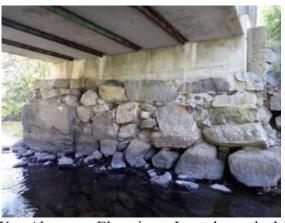
West Abutment Elevation – Loosely stacked stone with multiple gaps between stones. Note masonry portion collapsing at end of the abutment.
