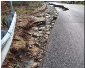
South Approach Roadway – Previous washout of roadway adjacent to bridge in December 2023 due to overtopping and flooding at the bridge.
