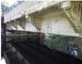
East shoulder supports with exposed rebar.
