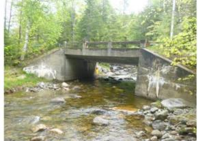
Southern elevation view. Note moderate cracks with efflorescence throughout.
