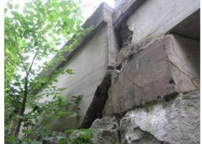
Southeast Return Wall – Shifted return wall, fascia girder with large spall at beam end, and cracks throughout fascia and concrete bridge seat.
