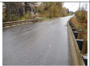
Top of Roadway Surface. Note cracks at the abutments.
