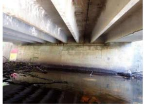
Underside of Superstructure – Evidence of leakage, rust staining, and scattered spalls between beams. Note scour placard on abutment.
