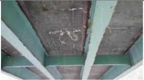
Deck Underside – Map cracking with efflorescence throughout. Note surface rust on top flanges of girders.
