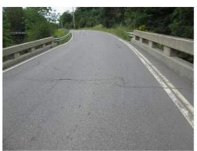
Top of roadway surface. Note crack in wearing surface.
