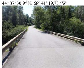
Top of Roadway Surface. Note settlement cracking at the abutment.
