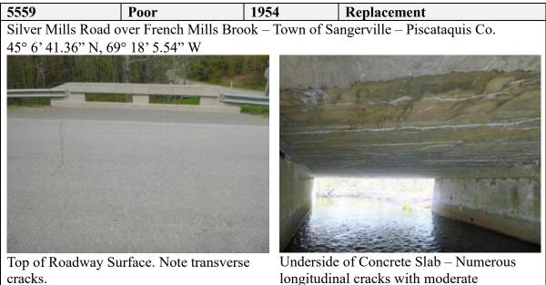
longitudinal cracks with moderate efflorescence build up.
